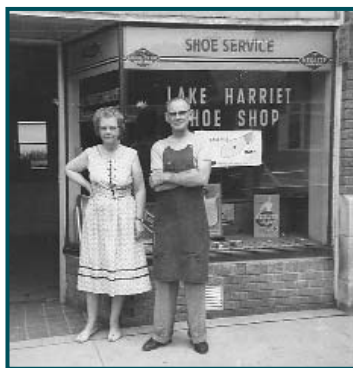
Ernie Lindstrom and his wife outside their shoe repair shop at 4302 Upton, ca. 1963 ▶
