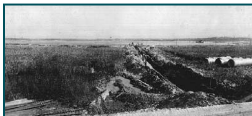
Storm sewer excavation at Lake Calhoun
