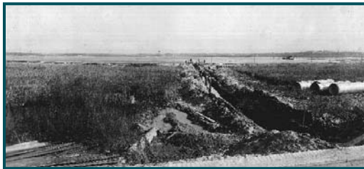
Storm sewer excavation at Lake Calhoun
