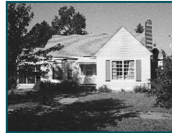
◀ 4256 Linden Hills Blvd., ca. 1990. The house pictured was elevated and incorporated into the second floor of the current house
