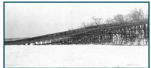
▲ A Park Board toboggan slide that originated at 42nd and Linden Hills Blvd. carried sliders down the hill onto the wooden structure and over the lower roadway and streetcar tracks. The lumber was salvaged from the courthouse at Bridge Square in downtown Minneapolis when it was demolished, ca. 1915
